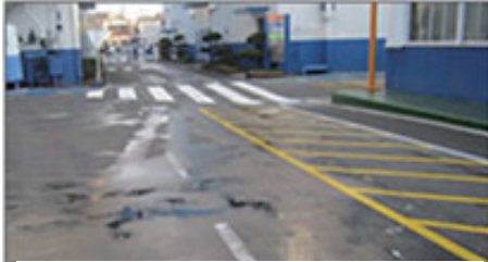
Headquarters: Oil leakage from delivery truck
