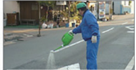
Applying oil processing agent
